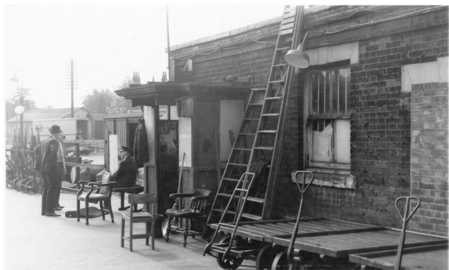
The north end of the old Platform 1 before rebuilding
