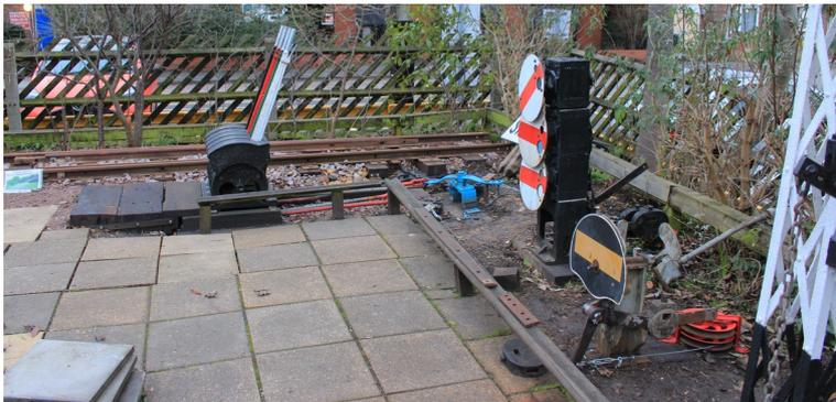
Left and overleaf: the new arrangement for the ground frame at the north end of the garden with the four levers now operating three signals and the ex-Talylyn points. Also pictured overleaf is the new Buffet building and the resited and elevated speed restriction termination sign.
