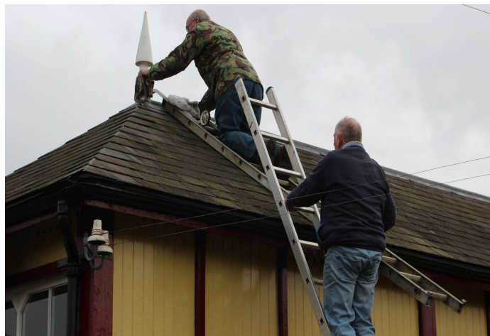
'Sherpa' Tony and John Telford repairing the finial at the north end of the 'box'.
