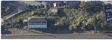
The signal box and grounds from the air
